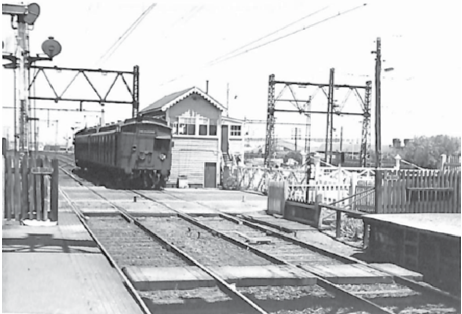
Graham Street Railway Gates - PMHPS
