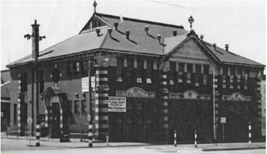
St. Joseph's Primary School, Port Melbourne cnr Rouse & Bay Streets - PMHPS
