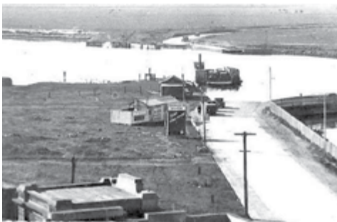
The 2 nd Williamstown Ferry operated from 1907 - 1931. Image shows the roads leading to the ferry - PMHPS
